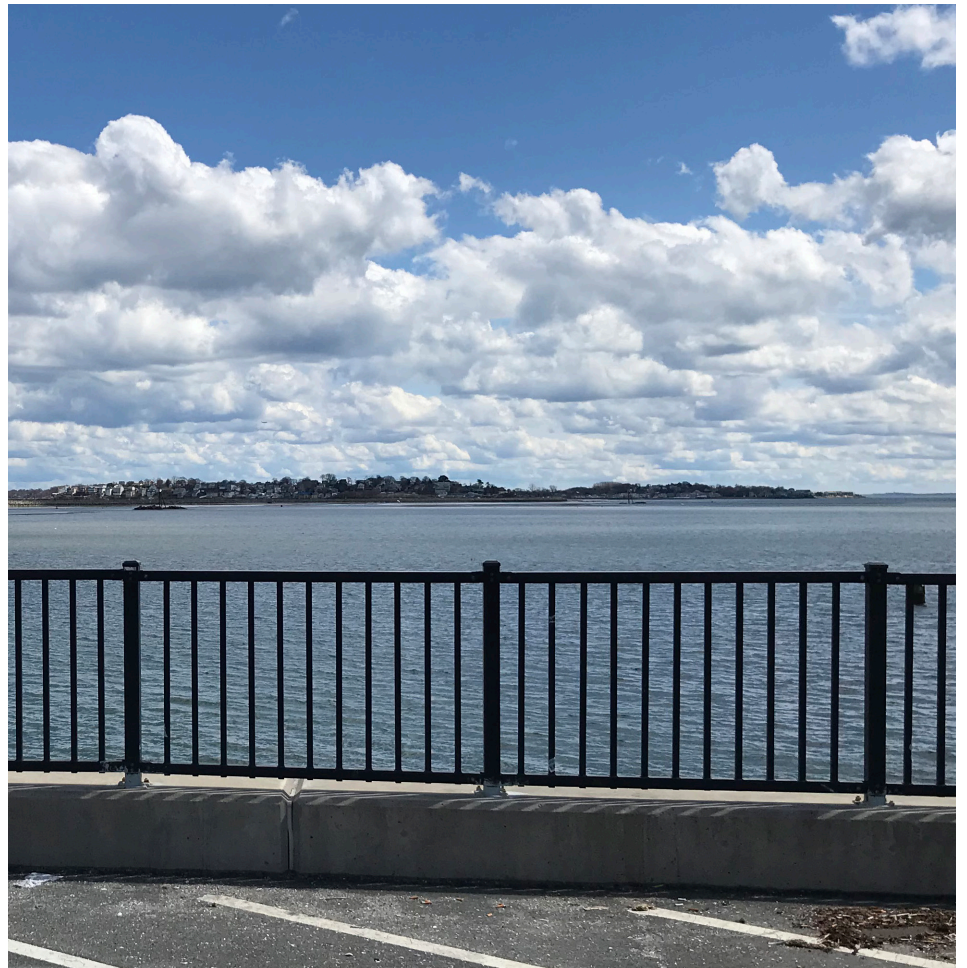
Top: Deteriorating timber bulkhead and eroding shoreline
